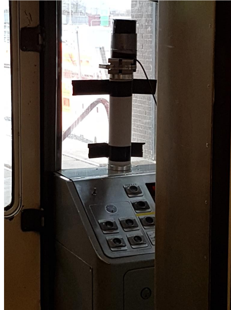
5G SA UE & Antenna inside unoccupied driver's cabin at rear of train
